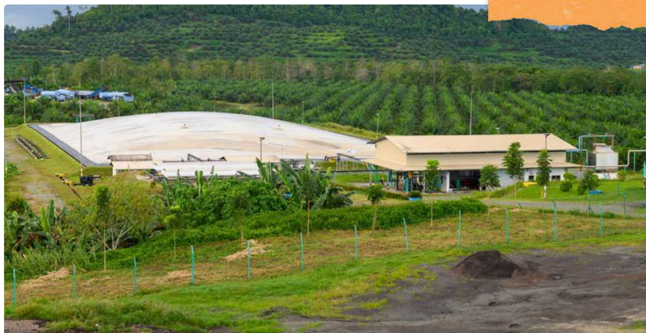
Methane capture plant in Sabahmas Mill, Malaysia.
