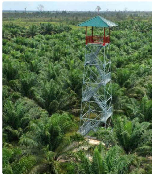
Observation towers are used for fire monitoring in Wilmar's plantations in Indonesia.
